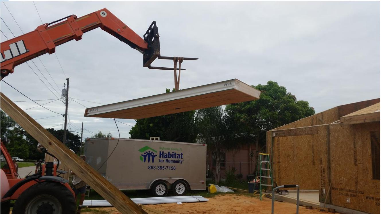
*Figure 3 - Here is the “LULL” starting to lift an 8' x 14' panel into position on the roof above the garage.*
