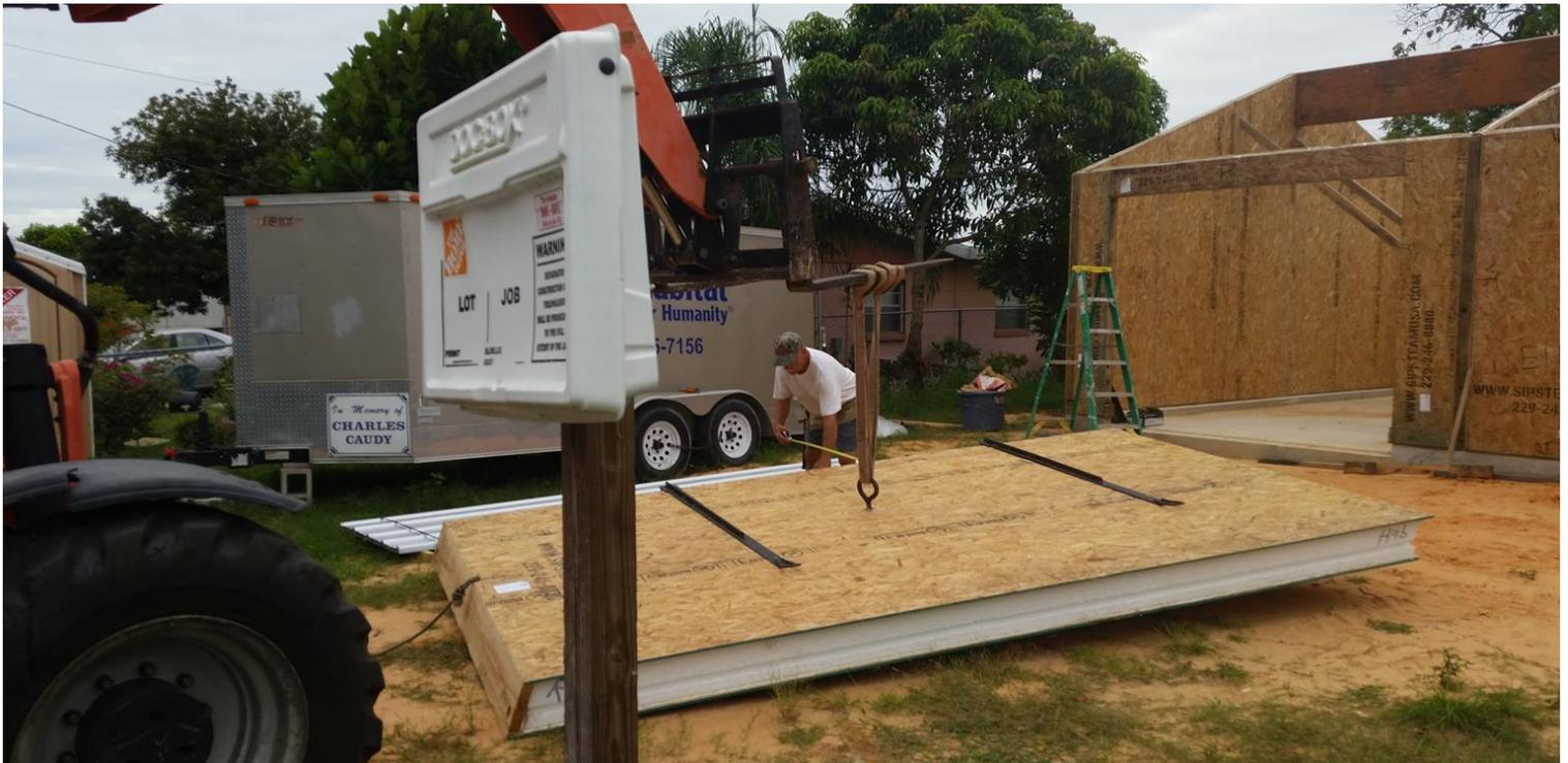
*Figure 2 - Getting ready to lift the 8' x 14' roofing panel*
