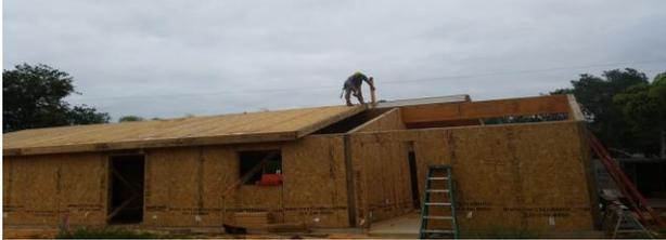
*Figure 7 - Here Frank is “adjusting” a roof panel into the correct position (with a sledge hammer and a 2x4)*
