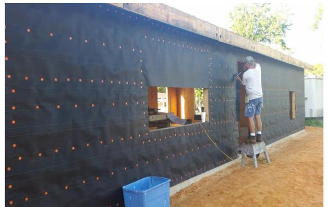
*Figure 11 - Buck replacing a non-perfect nail*
