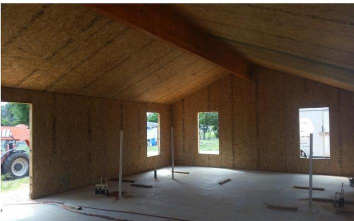
*Figure 8 - An interior picture of the assembled house*
