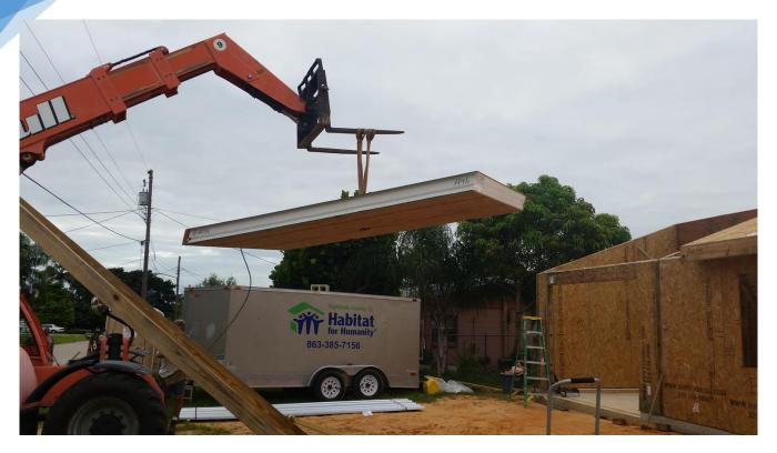
Figure 3 - Here is the "LULL" starting to lift an 8' x 14' panel into position on the roof above the garage.
